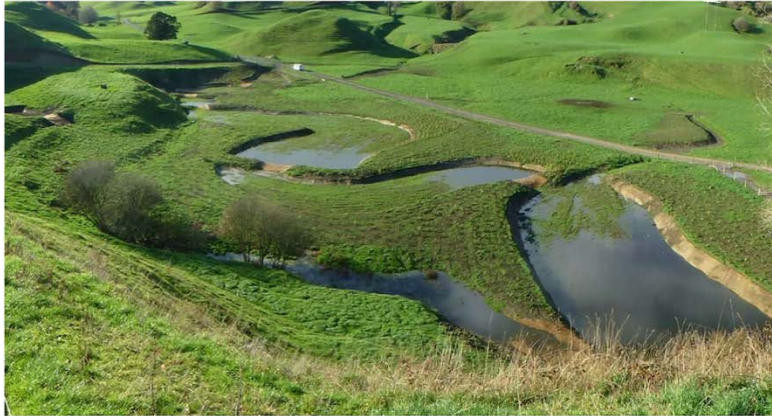
Figure 13: Example of a multi-cell wetland prior to planting. By creating multiple cells with a serpentine design, the bund height between cells is kept to a minimum. The design allows treatment of three major drain/stream inputs as well as runoff from the raceways. Use of curved edges to the wetland cells creates a natural appearance. Note also Figure 14.
