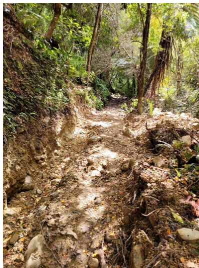
Figure 2 Pre Restoration of Donnelly Loop Track
