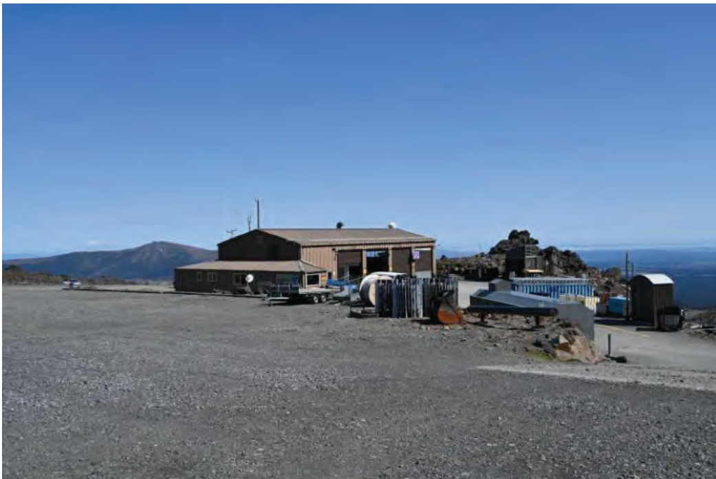
Figure 2: Lower maintenance workshop
