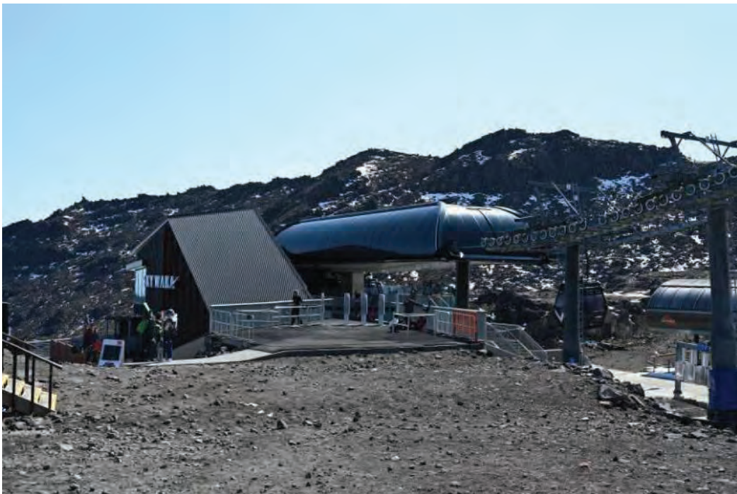
Figure 6: Sky Waka Gondola lower terminal building
