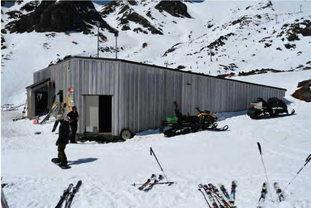
Figure 9: Knoll Ridge maintenance building
