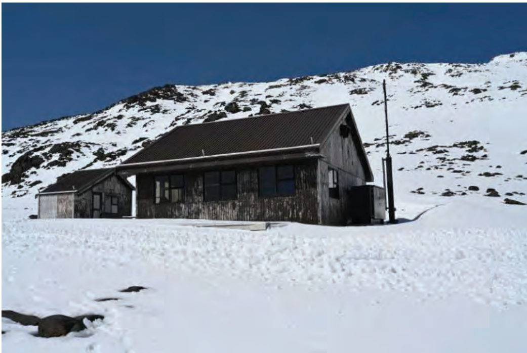
Figure 12: West Ridge buildings to be removed
