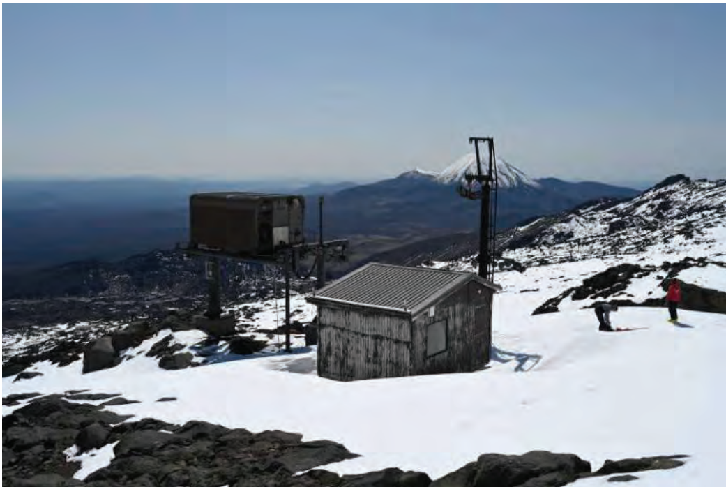
Figure 14: Far West T-bar drive terminal and operators shelter
