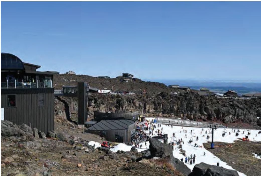
Figure 4: Sky Waka Gondola lower terminal building and Happy Valley infrastructure
