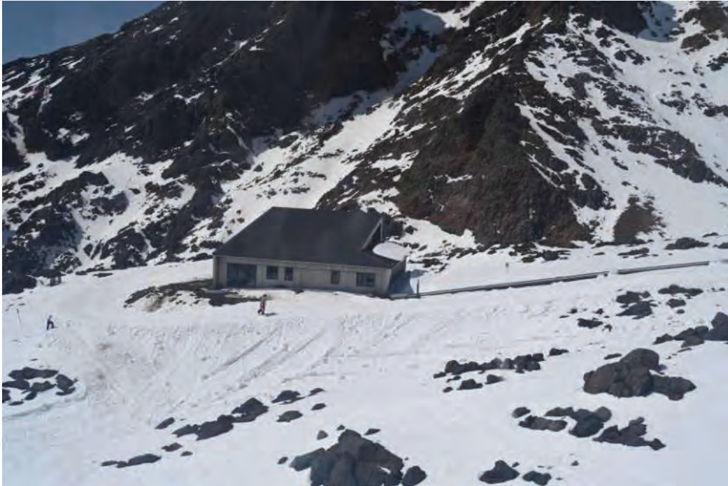
Figure 7: Snow groomer maintenance building
