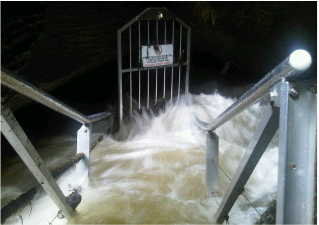
Figure 7 – Photo of the cave in flood
