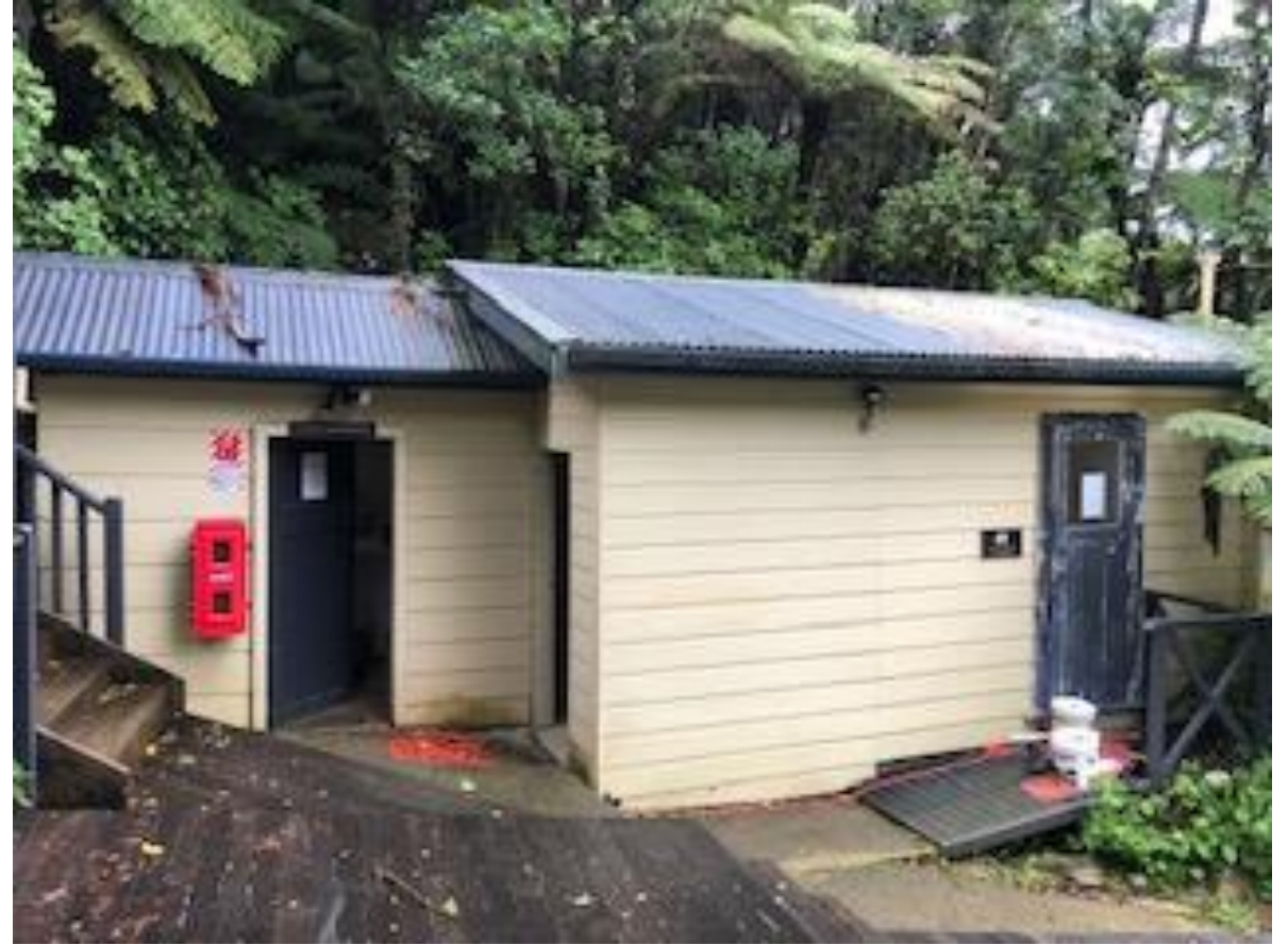
ANC12 Toilet & Shower Blk
