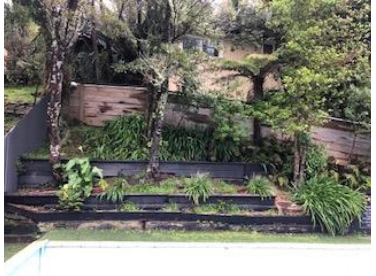
ANC6 Part - Pool Retaining walls
