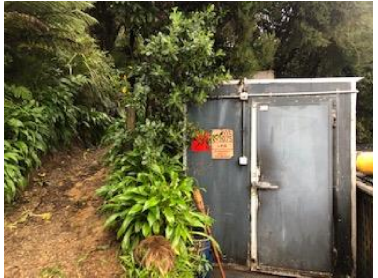
ANC 2 Part - Freezer Chiller
