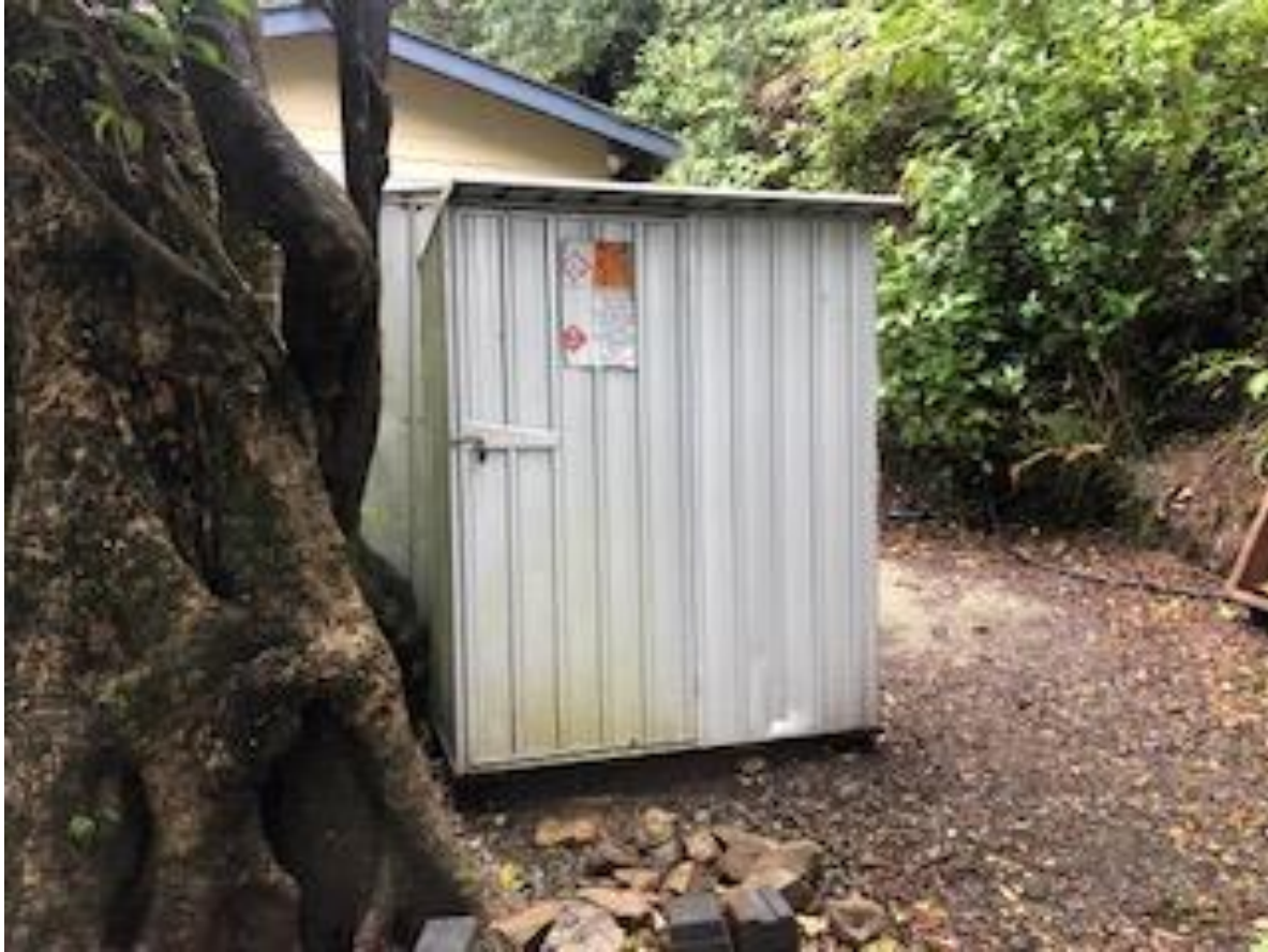
ANC13 - Gas Storage Shed
