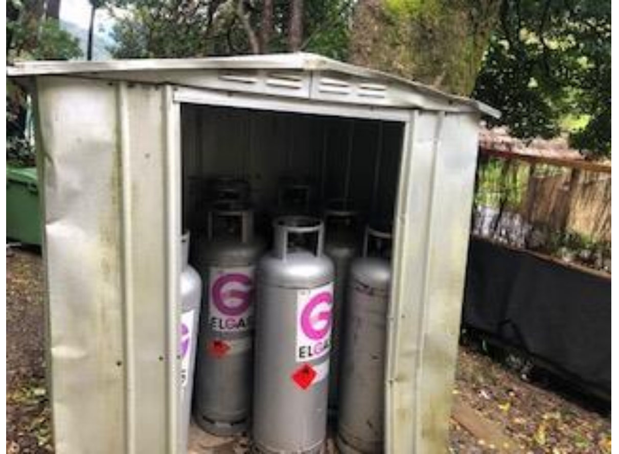
ANC13 Gas Storage Shed front
