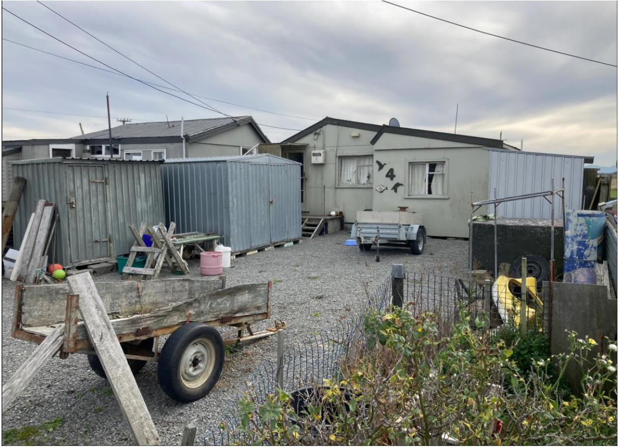
Hut 4 – Front view
