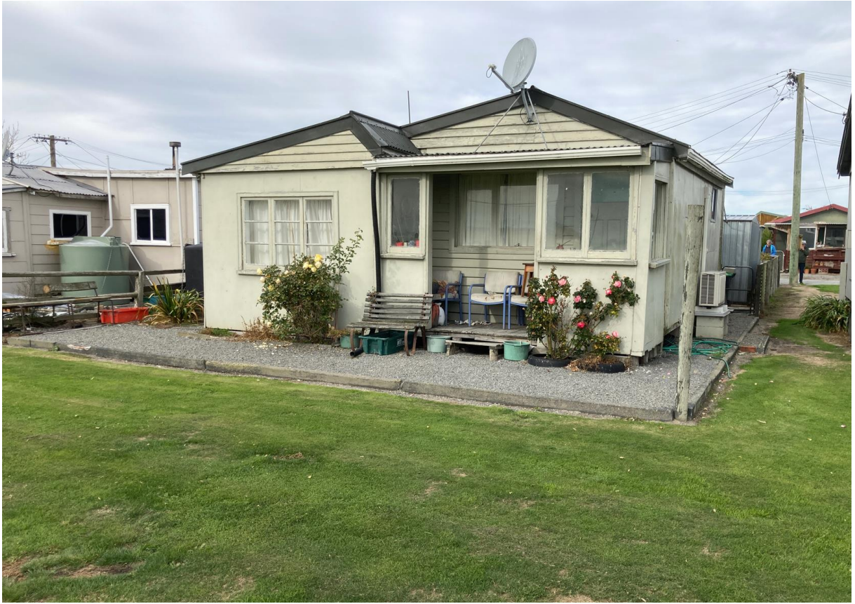
Hut 4 – Rear view
