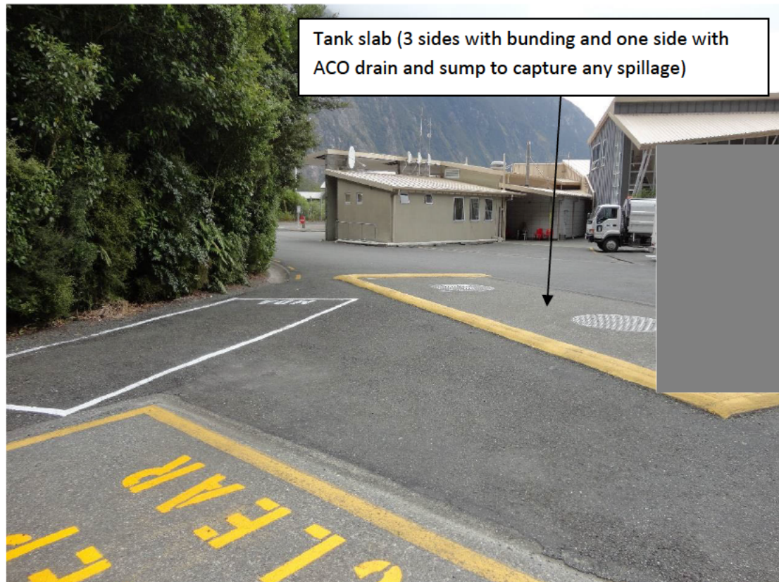
Photograph 2: Photo showing tank slab
