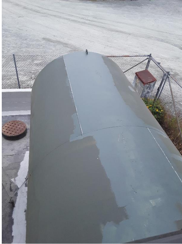
Photograph 3: Photo on top of the tank
