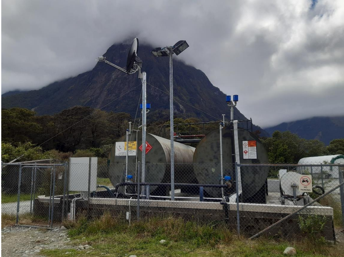
Photograph 1: Photo showing the tank compound
