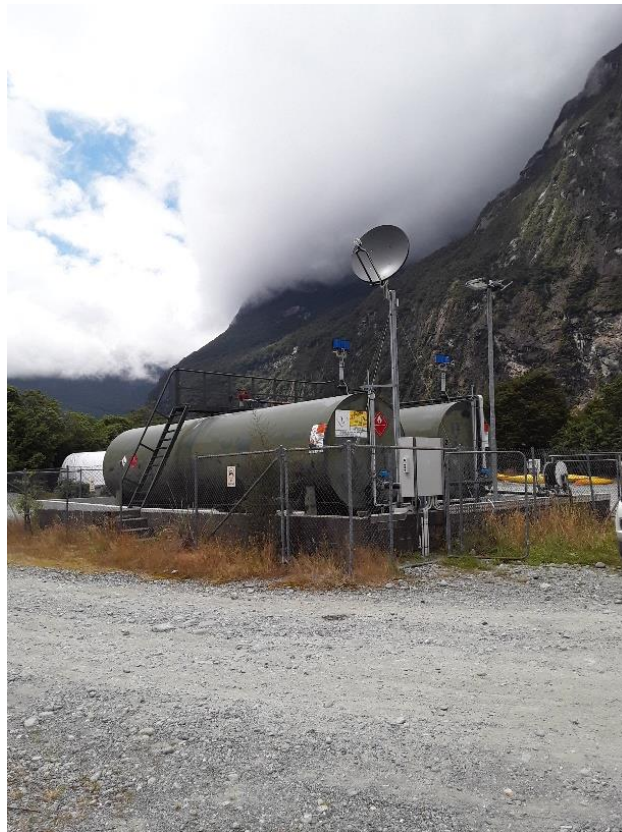
Photograph 2: Photo showing the tank compound
