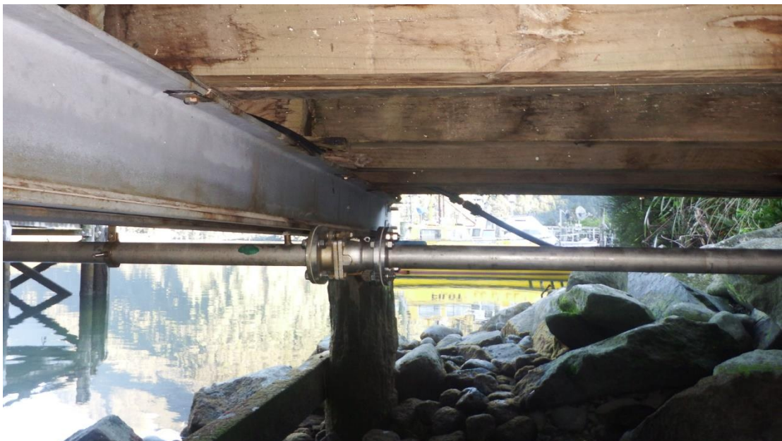
Photograph 6: Photo of the stainless-steel pipework beneath the wharf
