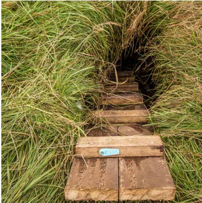
Figure A9.2 Single new ramp (K595) installed in 2015/16 at Sandy Bay on Enderby Island
