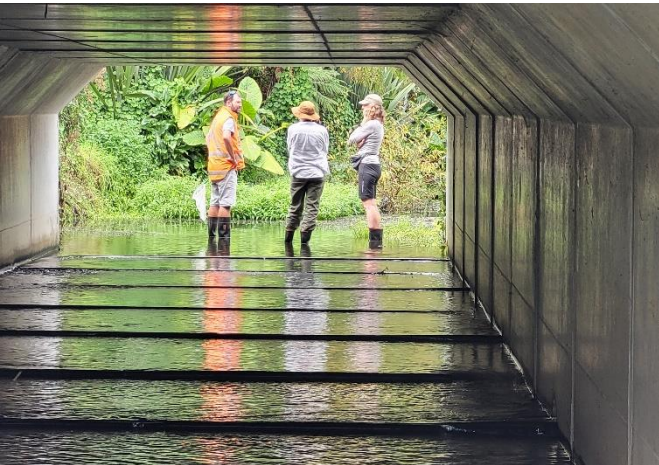
Flexible baffles across this culvert in a tributary of the Whanganui River have improved fish passage by slowing the water flow across its base. Photo: Carol Nicholson, DOC
