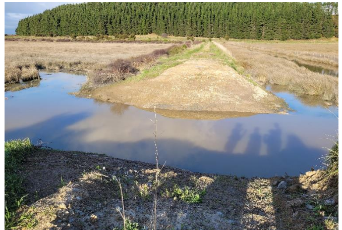
A gap created in this stop bank allowed fish to access the upstream wetland (left). Photo: Carol Nicholson, DOC
