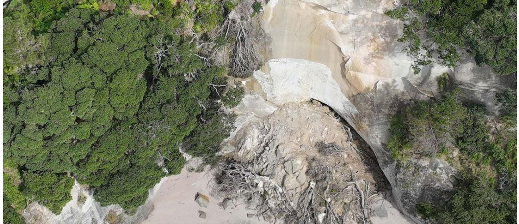
Photo: Slip at Cathedral Cove track. Image: DOC.
