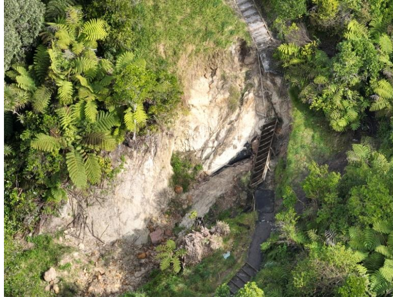
Image: DOC. Landslide and staircase slip at Cathedral Cove Track.
