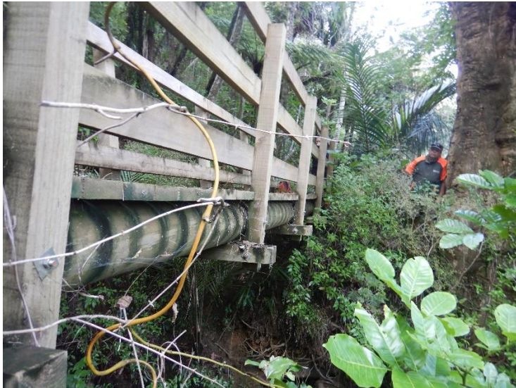
Figure 1: All pole bridges in good condition
