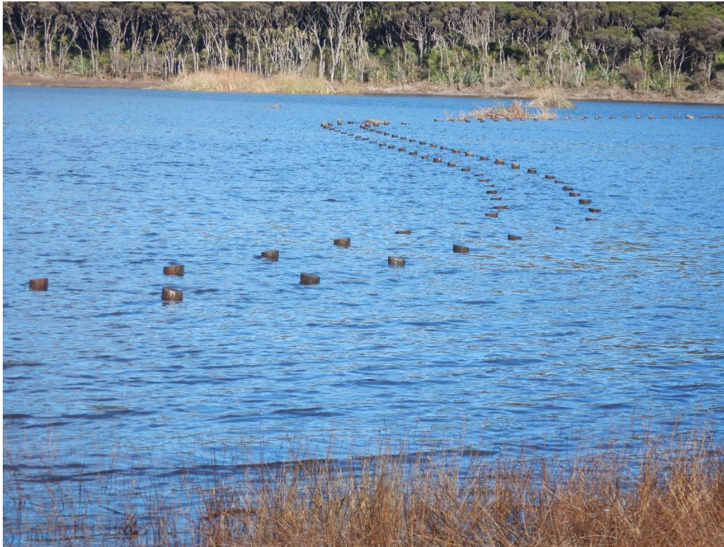
Figure 17: Waitahora lagoon boardwalk at the time of inspection 12.44pm 25 May 2023. Water depth over the boardwalk deck approximately 0.5m.
