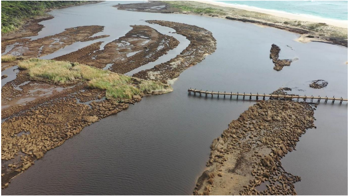
Figure 16: Drone view of Waitahora Lagoon Boardwalk in mid May showing missing 10m section.
