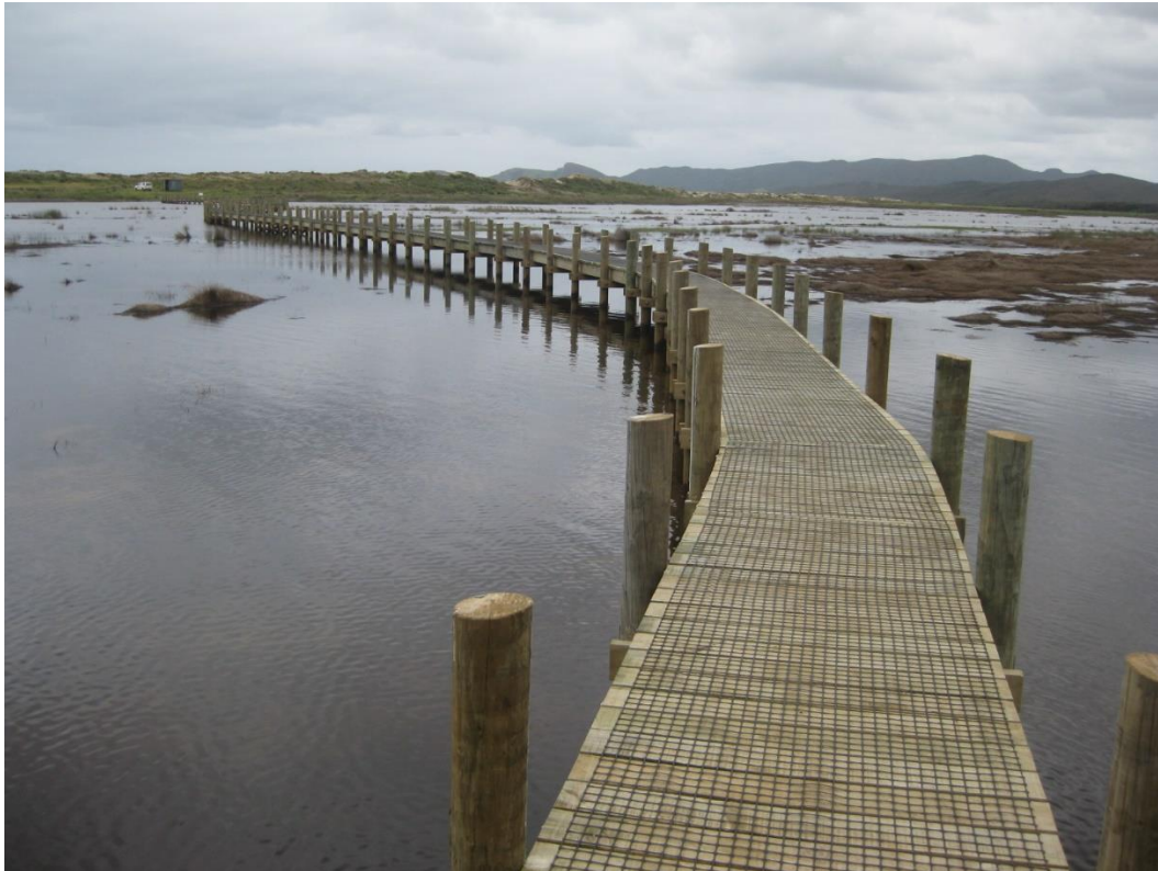
Figure 16: Waitahora lagoon Boardwalk soon after completion in 2012
