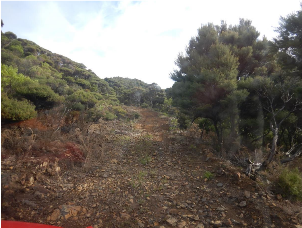
Figure 5: Surface water is bypassing drainage cut-outs
