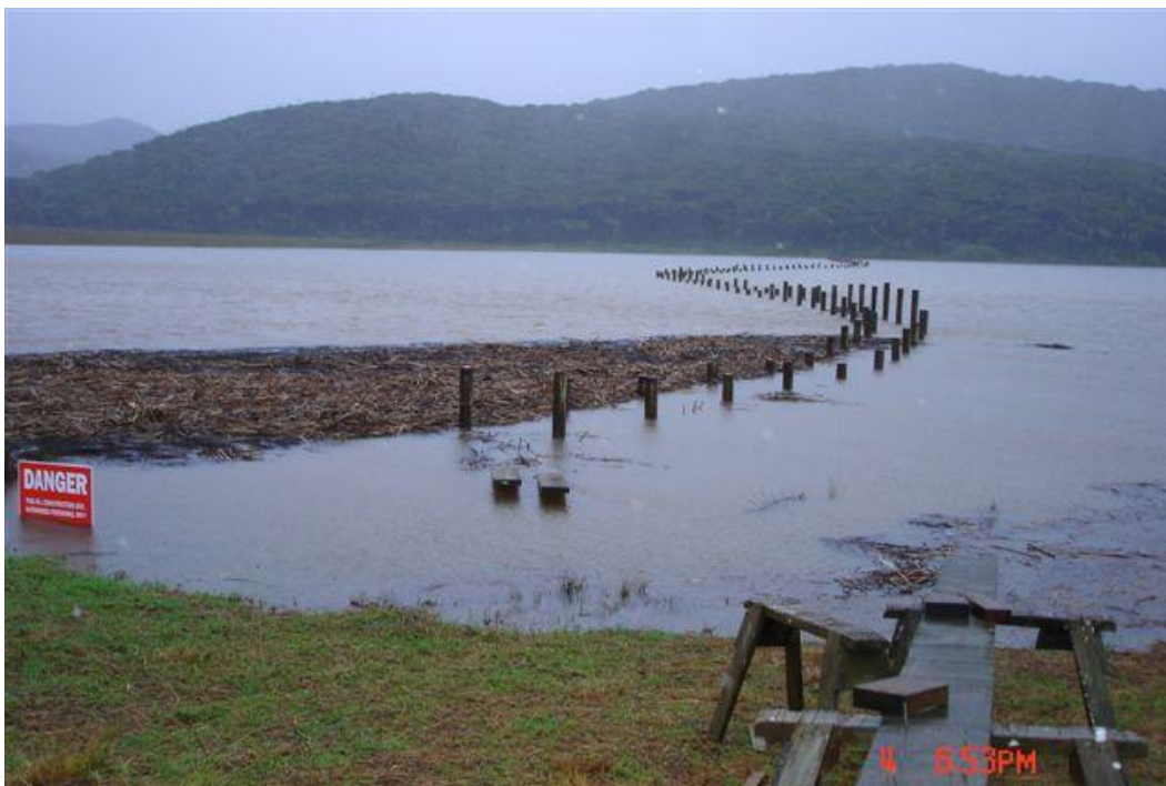
Figure 15: Waitahora Lagoon Boardwalk inundated during construction. Note raised piles and accumulated debris.
