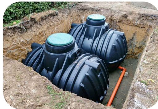
Toilet Waste Monitoring
