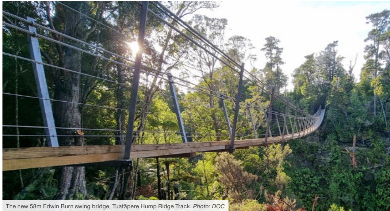
The new 58m Edwin Burn swing bridge, Tuatāpere Hump Ridge Track. Photo: DOC
