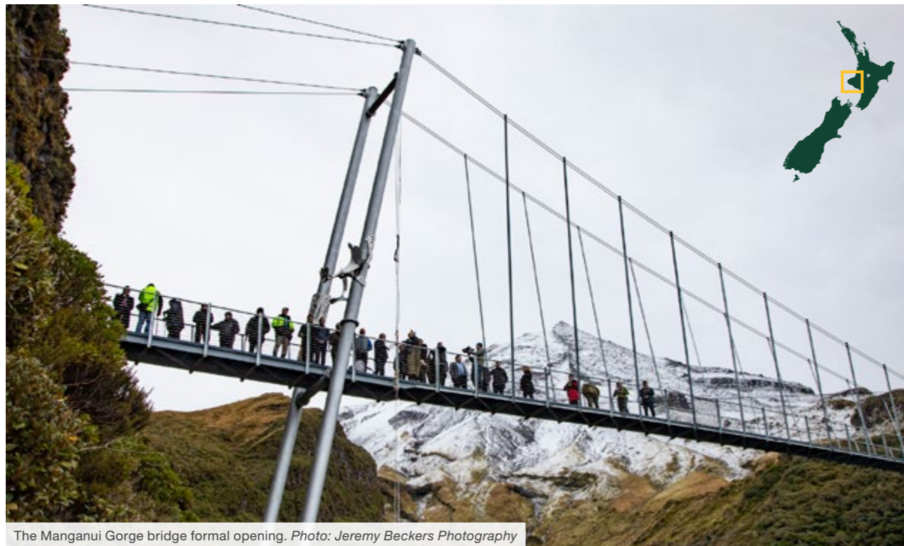
The Manganui Gorge bridge formal opening. Photo: Jeremy Beckers Photography
