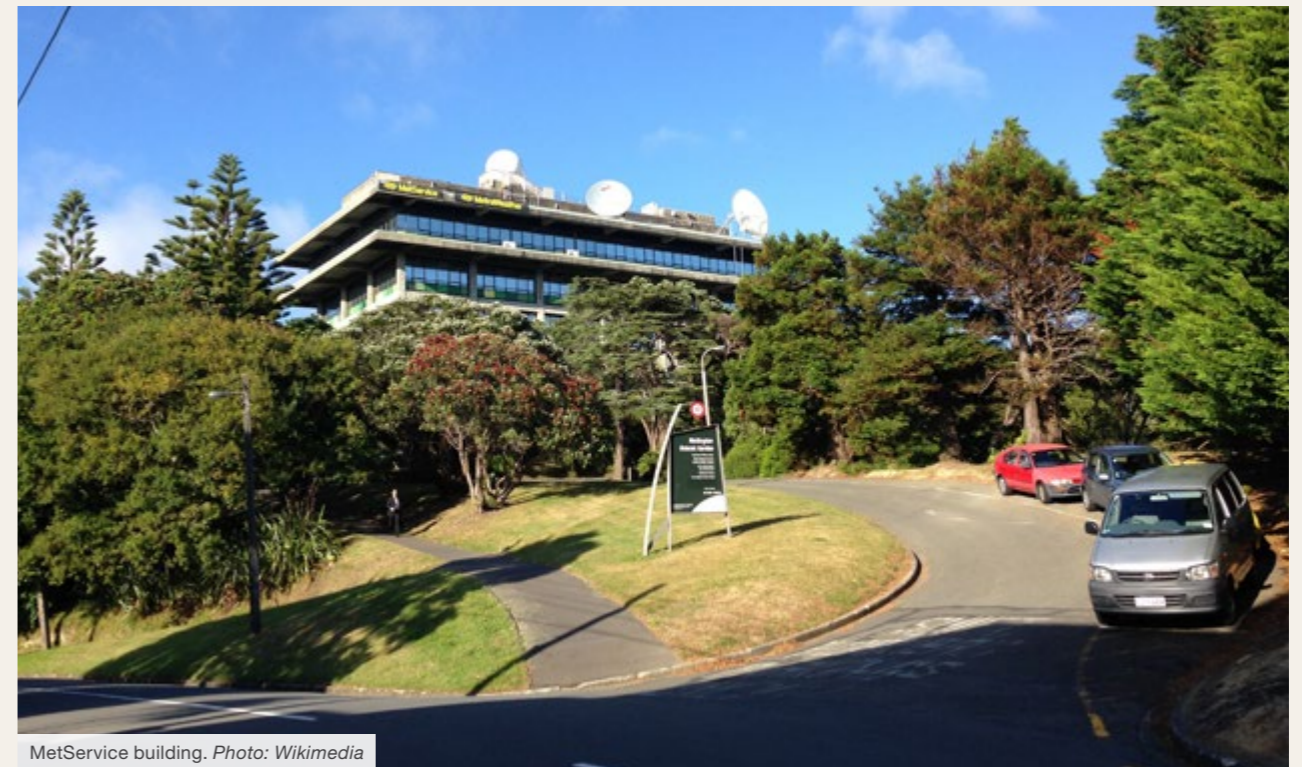
MetService building. Photo: Wikimedia
