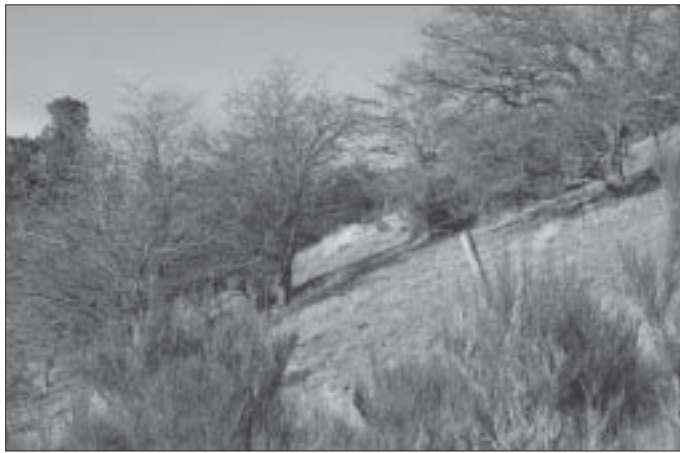
Figure 12. View across hill slope above subject buildings. Fence post is normal to the c. 25° slope.
