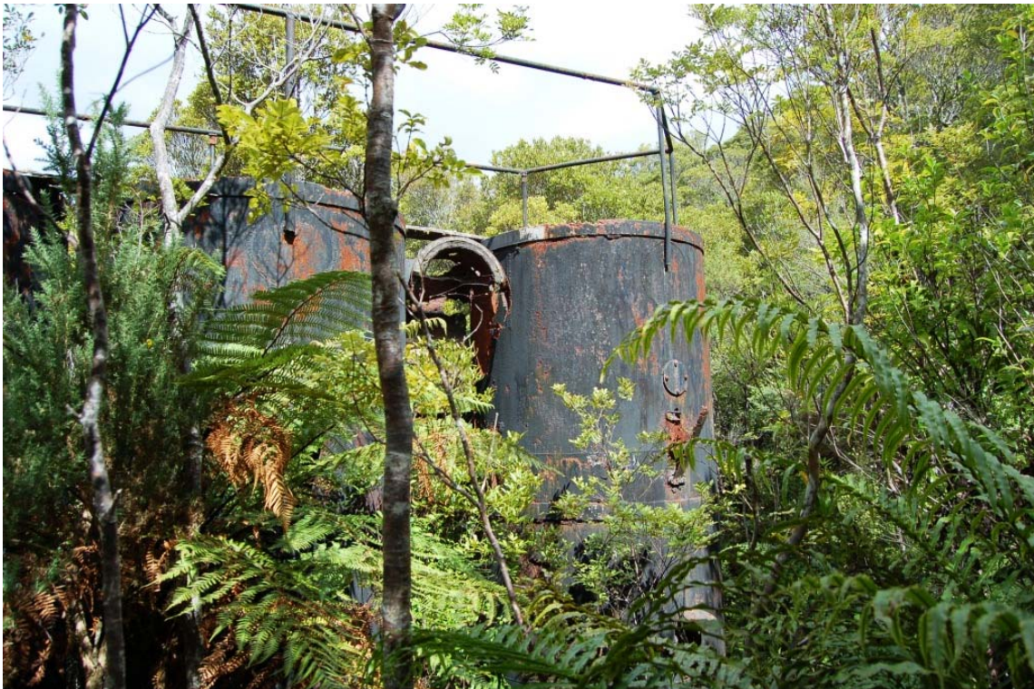
Figure 7: Towers. Above: Southern aspect of towers in 1968. Note handrail around the top and large inlet pipes connected to the “exchange” by way of terracotta pipes. Photo from the collection of Anne and Brian Reed. Below: Northern aspect of towers in April 2010. Note the large “outlet” pipe.
