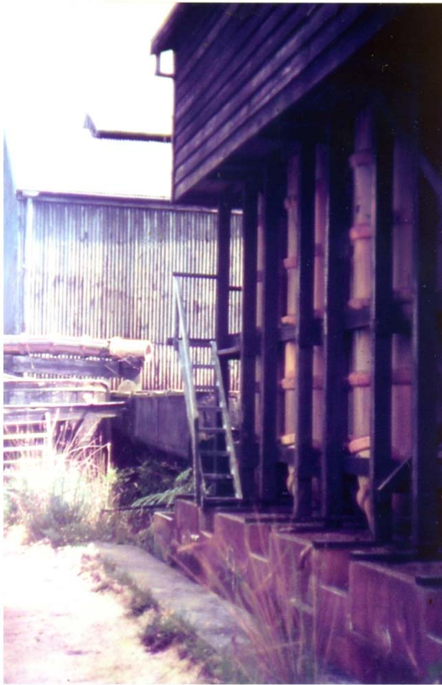
Figure 8b: The Pipe Battery in 1968. Evidenced today by a series of low concrete troughs, visible at the bottom of this photo. This photo was taken facing the south, looking back at the corrugated iron building which housed the furnace. The “cooling trough” (G) is visible behind the ladder.
