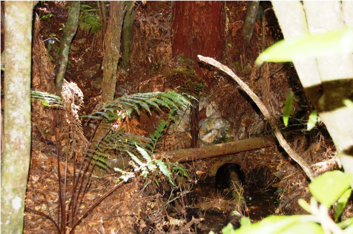
Figure 2: Looking down the channel below the dam, note that the iron pipe continues for some distance down the stream (left); the culvert and pipe set into the bottom of the dam (below).
