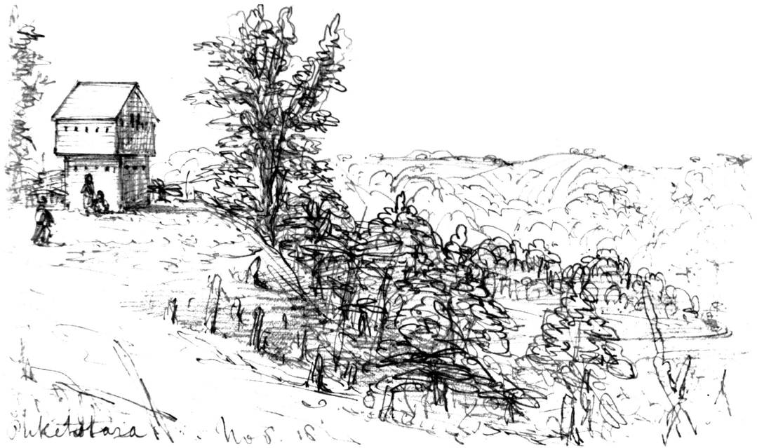
Figure 9. 'Puketotara Nov. 18' [1864]. Puketotara Blockhouse (9.22), near New Plymouth, is an example of a two-storey work. Colonel H.J. Warre, Sketchbook 1864-1865, p. 51, Ref: E-294-051, Alexander Turnbull Library, Wellington.
