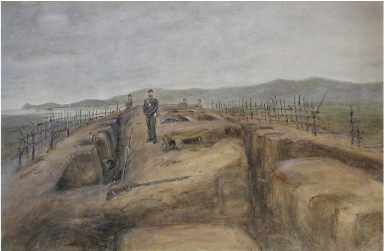
Figure 14. Pukehinahina/ Gate Pā (5.11), showing the slight fence and small pā interior, and traversed firing trench with access to underground bunkers. Lieutenant H.G. Robley, 68th Regiment, watercolour, Auckland Museum PD48(47).
