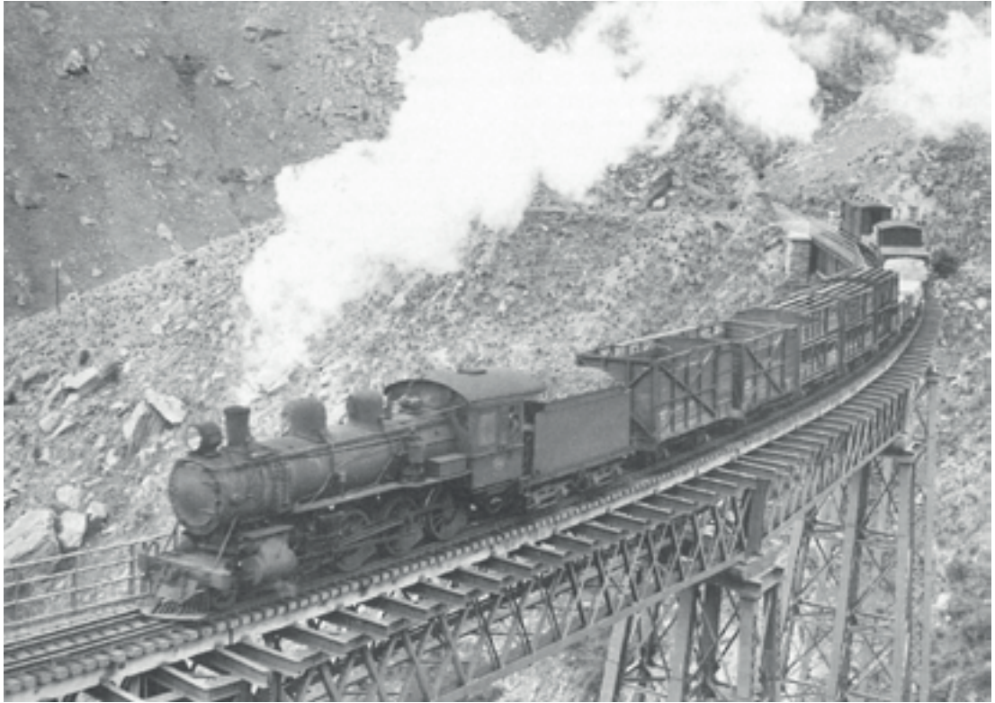
Figure 9. Economic operation of the Otago Central Railway was bedevilled by small steam locomotives and short trains. From 1910 to 1940, the principal locomotive class was the 36-ton Ub, capable of hauling only 160 tons. This train of 12 wagons included 5 stock wagons at the front. Even the ultimate step-up to the 53-ton Ab class allowed only 240-ton trains – trains needed to be twice that size to be profitable. Taken in May 1937 on the graceful curved Flat Stream Viaduct in the dramatic Taieri Gorge. Photo: Stan Rockliff, J.D. Mahoney collection.
