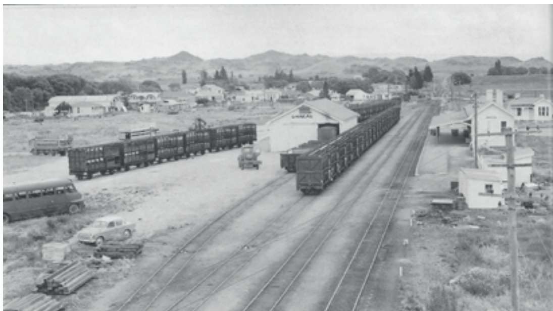
Figure 15. Omakau overview. This scene demonstrates the scale of sheep traffic at Omakau. In January 1968, this seasonal traffic is at its peak, with over 40 sheep wagons being loaded. At Omakau station, the purpose of most of these sidings is to facilitate this traffic. The traditional stockyard sidings are on the upper right. An additional sheep loading siding on the left was installed in the mid-1950s to allow direct loading from road vehicles. In the days of steam locomotives, 40 wagons would constitute a whole train that originated most days in the peak season from Omakau. This busy scene would soon be history – just 5 years later in 1973, railways would cease hauling stock. Photo: George Emerson.
