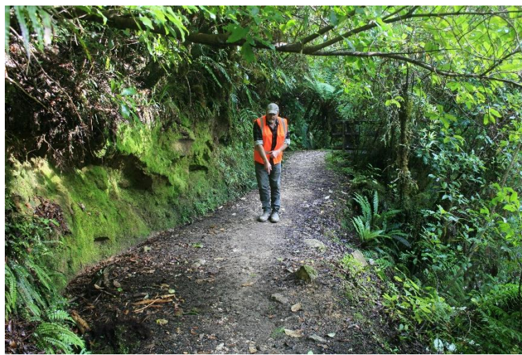
Figure 8 Ōpārara track; Upgrades here include relocating the track surface to the left of the figure to avoid undermining currently occurring downhill of the track. The retired section of track bench will be revegetated. Photograph by J.Head 6 August 2020.
