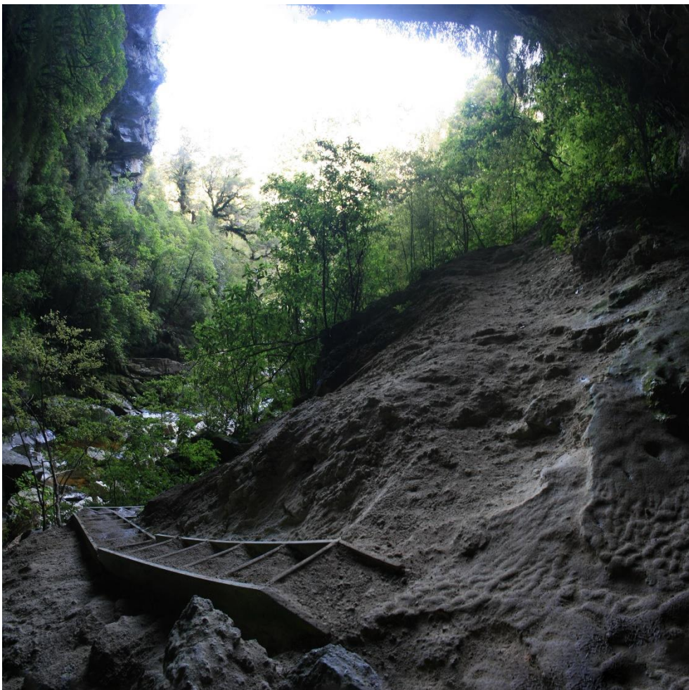
Figure 14 View from the end of the Ōpārara track at/under the arch. The mattress will be placed over the limestone bedrock to provide a level surface and protect the rock (at lower right/top of stairs). The timber stairs will be removed. The new track will enter the arch near the top right of the photograph. Photograph by J.Head 6 August 2020
